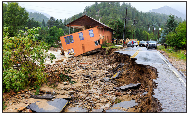
Flooding from heavy rains damaged Boulder, Colorado, in September 2013—one of several extreme events examined in the collaborative report. (Source: S. Zumwalt, FEMA)
