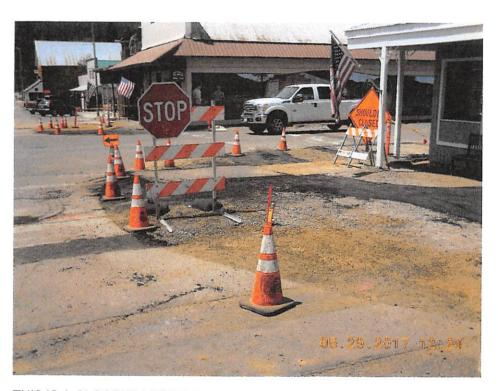
THIS IS A CLOSEUP VIEW OF THE MAIN STREET SPACE TO BE TAKEN UP BY THE TRAFFIC BARRIER/ISLANDS AT ALL FOUR CORNERS OF THE INTERSECTION. THEY PROTRUDE OUT INTO HIGHWAY 89 AS WELL AS MAIN STREET. IF THE INTERSECTION STREETS ARE LOWERED BY 18 INCHES, THE ENTRANCES TO THE BUSINESSES WILL BE 2 FT' HIGHER THAN STREET LEVEL. THEN THESE TRAFFIC ISLANDS WILL BE NECESSARY TO INSTALL ELABORATE
