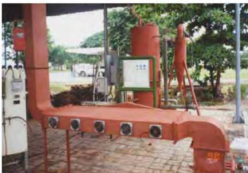
Figure 3.3: Biomass stove-heat exchanger unit without insulation
