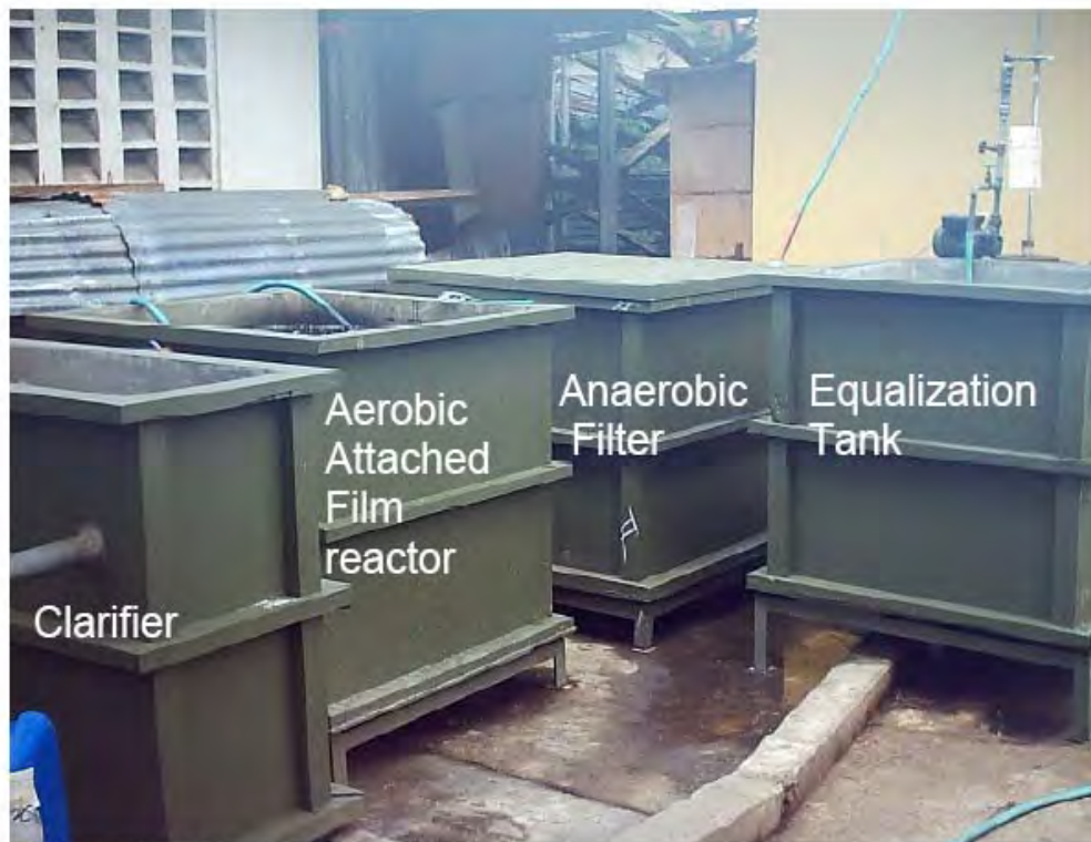
Figure 3 The pilot plant setup
