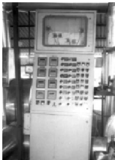
Figure 2. Programmable Logic Controller (PLC)-based control System
